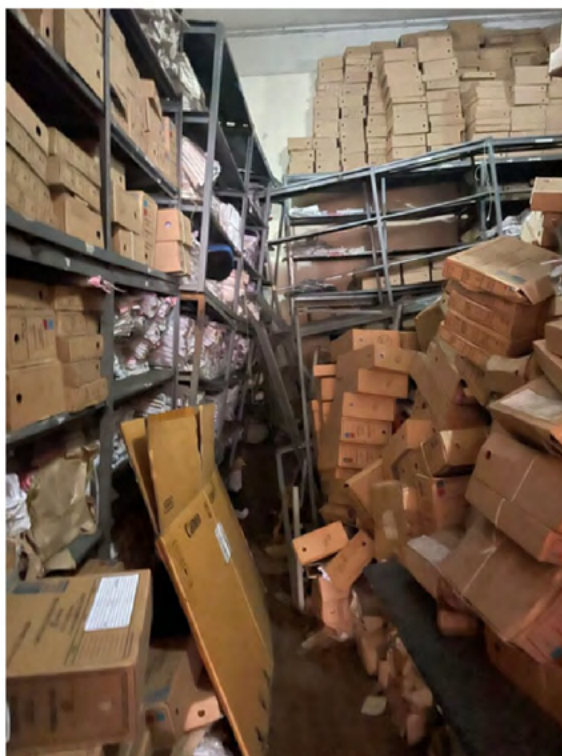
Figure 3: Too weak and overloaded shelves in the archives room of the SAI of Madagascar Source: Cour des comptes Madagascar
