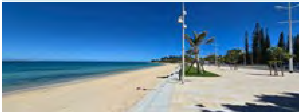
Anse-Vata Beach, April 2024, after consolidation works involving a reinforcement structure consisting of a concrete wall in the form of steps and an enlargement of the beach by removing the earth.
