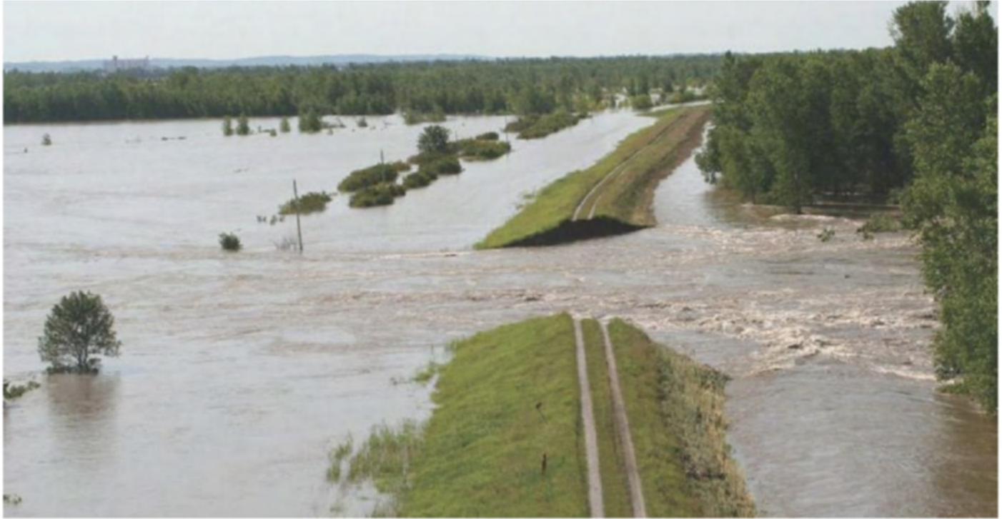
Figure 2: Breached Levee along the Missouri River, June 2011
